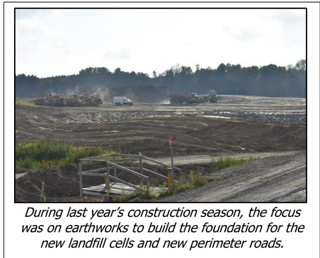
*During last year's construction season, the focus was on earthworks to build the foundation for the new landfill cells and new perimeter roads.*
