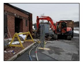
• The Gaseous Chlorine System at Warneck Pump Station, used to treat wastewater, was removed and replaced with a different type of treatment. This has greatly reduced potential danger to worker safety and residents in the area
